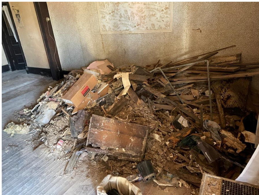
Photo 2. Pile of Debris with asbestos containing transite panels. Location: Dining Room
