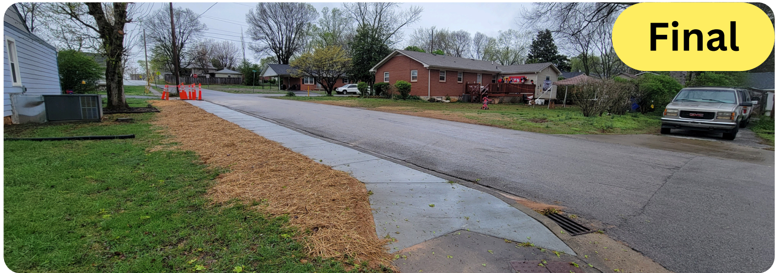
The Public Works Operations cement crew replaces old sidewalk at Liberty Way and Glendale Ave. The sidewalk was reported by a citizen as a tripping hazard. (Week of 17 March)
