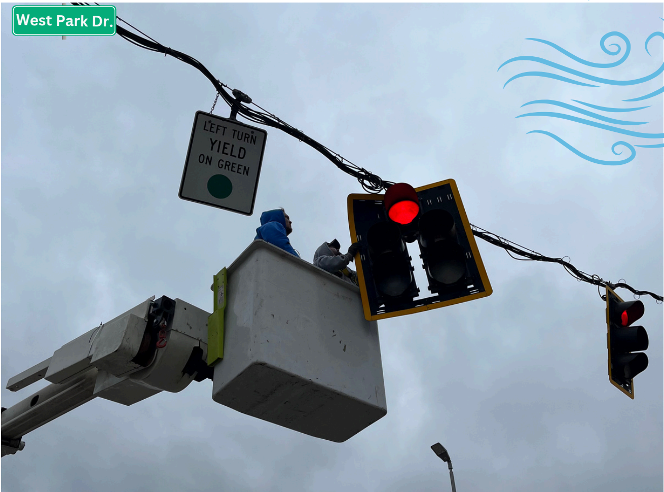
Signal Technician II Eric Joiner and Operations Maintenance Technician III Matt Barrow untangle a street signal caused by high winds at West Park Dr and Gary Farms Blvd (5 March).
