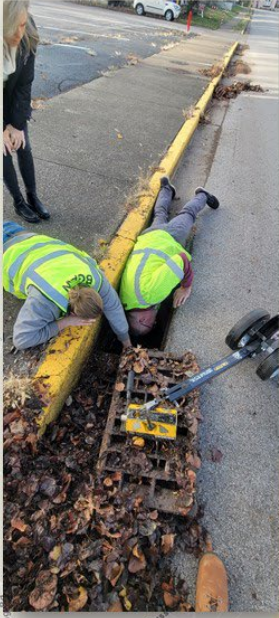
Elm St. & E. 10 th Ave Storm Drain Inspection Conducted: 5 Dec
