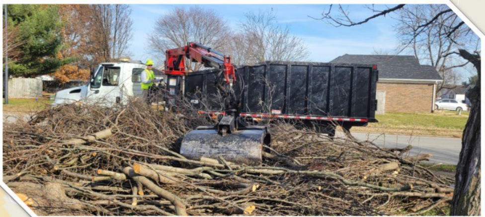
Fieldstone Farms Storm Debris Removal from RoW Completed: 13 Dec
