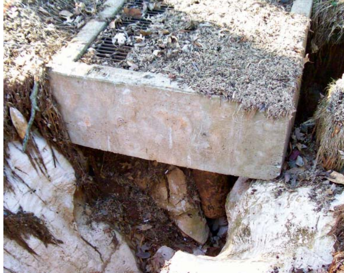
Soil collapse around drainage well
