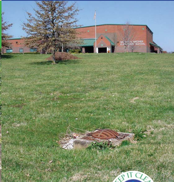
Soil collapse around drainage well
