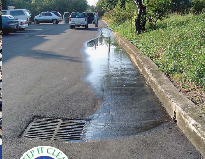
Leaking sewer line flowing into drainage well
