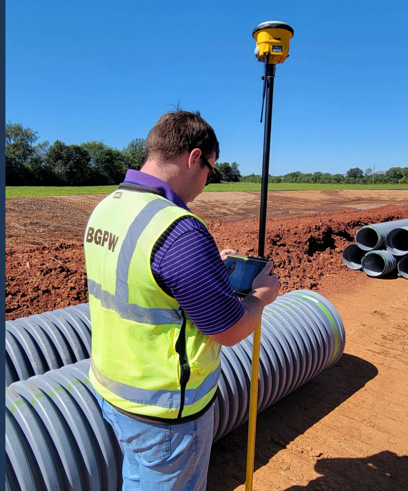
Surveyor I Tyler Phelps measuring the depth of the cut to finish asphalt grading at Bluegrass Farms Blvd. Extension Project. (October 10, 2024)
