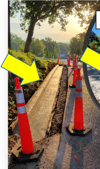
Figure 4-Curb and Gutter replacement along Parkway St (14 June)
