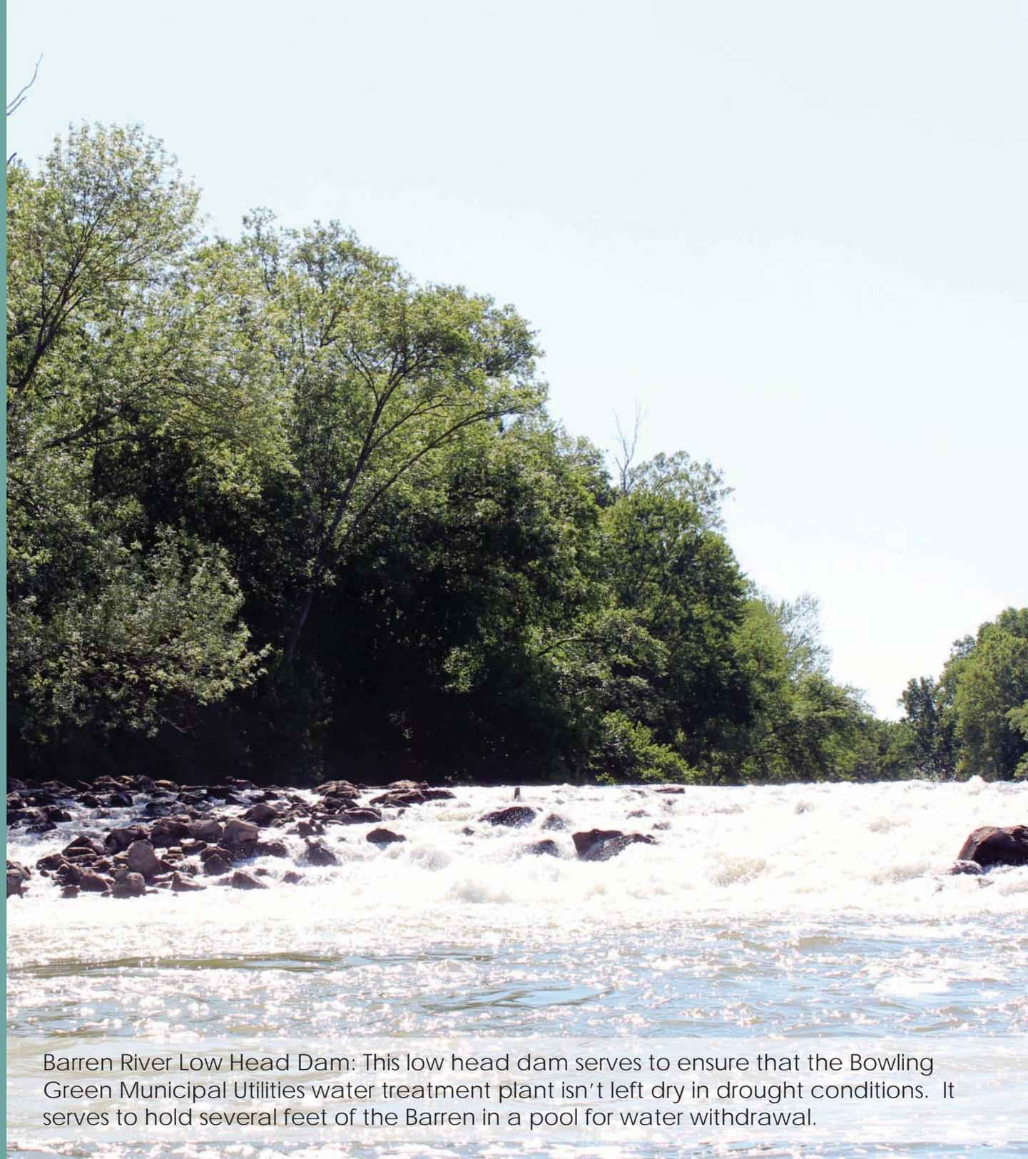
Barren River Low Head Dam: This low head dam serves to ensure that the Bowling Green Municipal Utilities water treatment plant isn't left dry in drought conditions. It serves to hold several feet of the Barren in a pool for water withdrawal.
