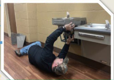
Water Fountain Maintenance BGPD (7 March)
