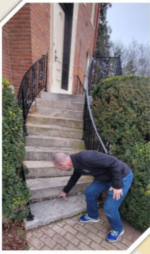
Stairway Inspection Hobson House (7 March)
