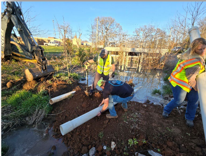
Figure 10-As contaminated water flowed from the Valor Oil Fire site, Public Works crews created a temporary underflow dam to prevent oil and gas from reaching the Barren River. They were assisted by crews from the Kentucky State Transportation Cabinet and additional pipe was supplied by BGMU. Environmental Manager Matt Powell, Environmental Coordinator Nick Lawhon and Construction Coordinator I Dara Price install pipe to allow clean water to flow and restrict contaminated water at the Whiskey Run storm outlet. (27 March)
