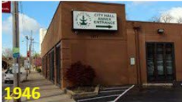
1946 City Hall Annex
