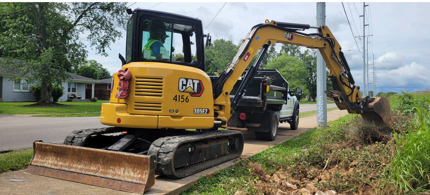
Operations Maintenance Technician II Austin Jones clears a drainage ditch along the City greenway near Creason Street , helping maintain proper stormwater flow and reduce localized flooding. Public Works' drainage crew responds to sinkholes, clears ditches and drainage channels, and installs Class V injection wells that help convey stormwater into Bowling Green's underlying karst system. (22 June)
