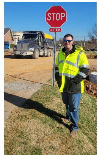
Figure 6-Construction Coordinator II Tyler Phelps oversees construction at the Westen St. and Patrick Way Roundabout (29 Nov)
