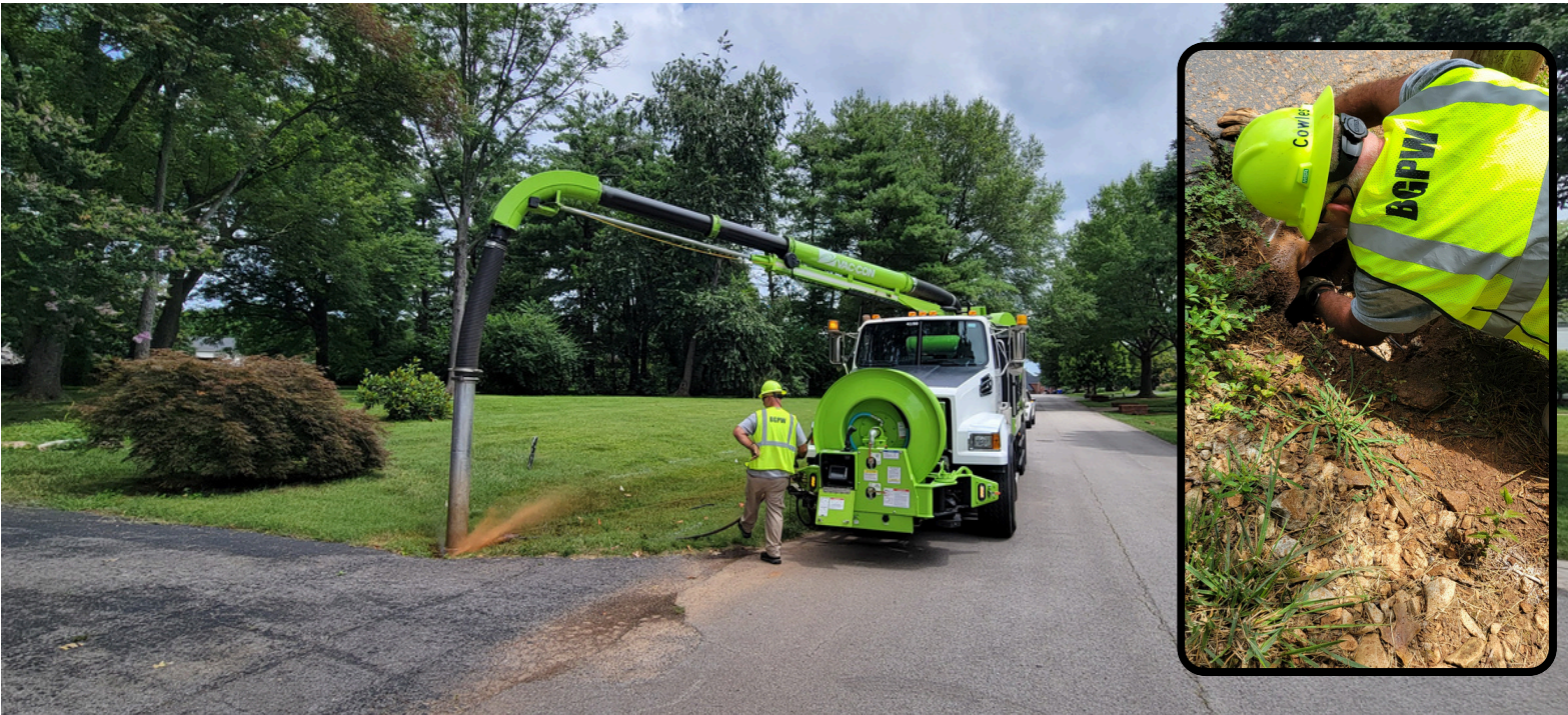
Operations Maintenance Technician III Timmy Cowles cleans a storm tile along Newberry Street. Drains, ditches and tiles are inspected and cleaned regularly across the city to help alleviate flooding. Fun Fact: Timmy’s record for a cleanout is 17 basketballs. On this day, it was 2 skunks. (7 July)
