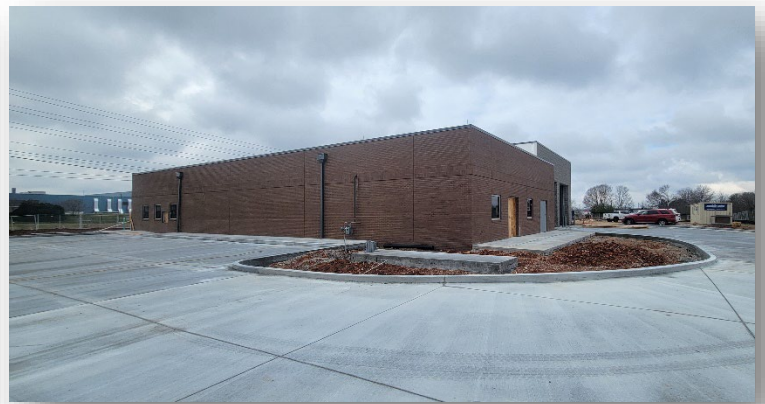
Figure 15-Facilities Manager Dave Hehner oversees construction progress at Fire Station #8. (31 Jan)
