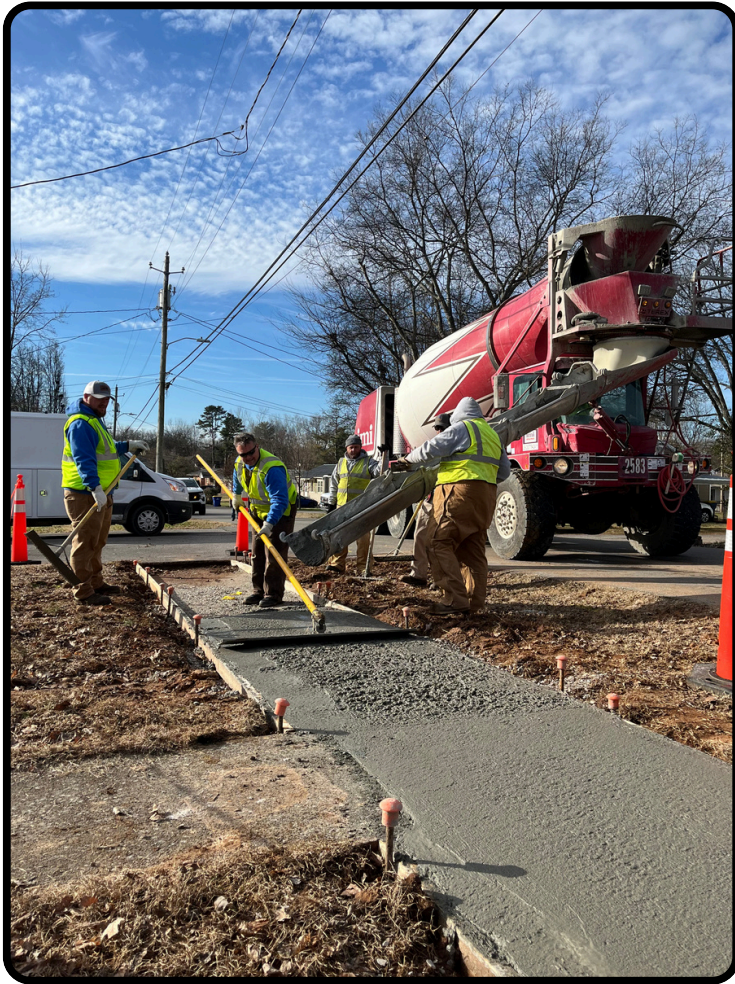
(Top) This month, our concrete crews have been actively engaged in pouring a new footer for an upcoming art sculpture in Circus Square Park, located at the intersection of E. 7th Ave and State Street . (Bottom) Despite facing inclement weather, the team successfully continued their efforts to repair and pour new sidewalks along Kirby Drive .
