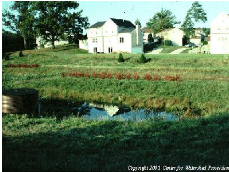
Figure PTP-03- 7 Micropool Extended Detention Pond.
