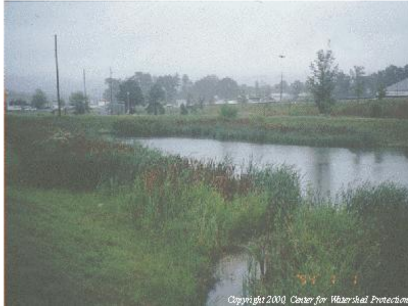
Figure PTP-03- 4 Wet Extended Detention Pond.
