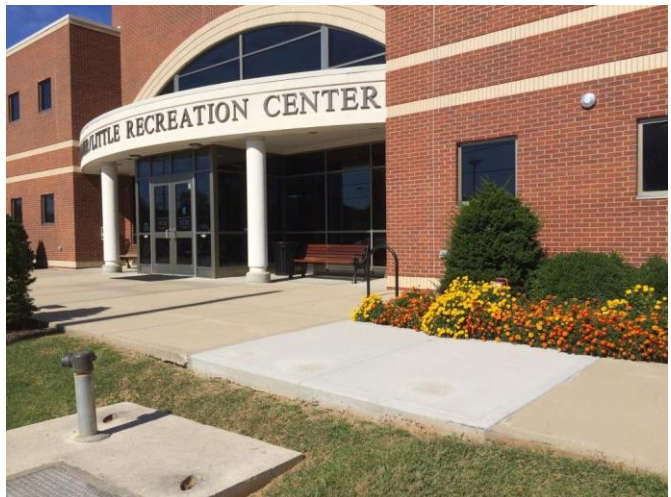
Sidewalk repair at Kummer-Little eliminated trip/fall hazard.
