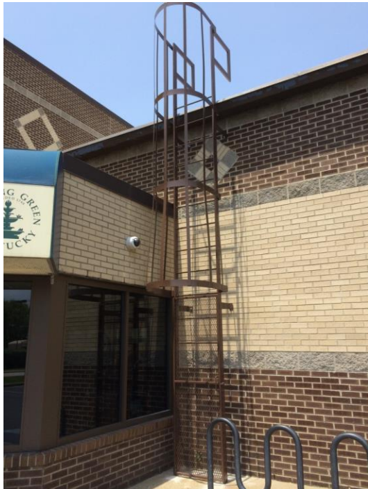
Fixed Ladder at F.O. Moxley Recreation Center provides safer access to roof.
