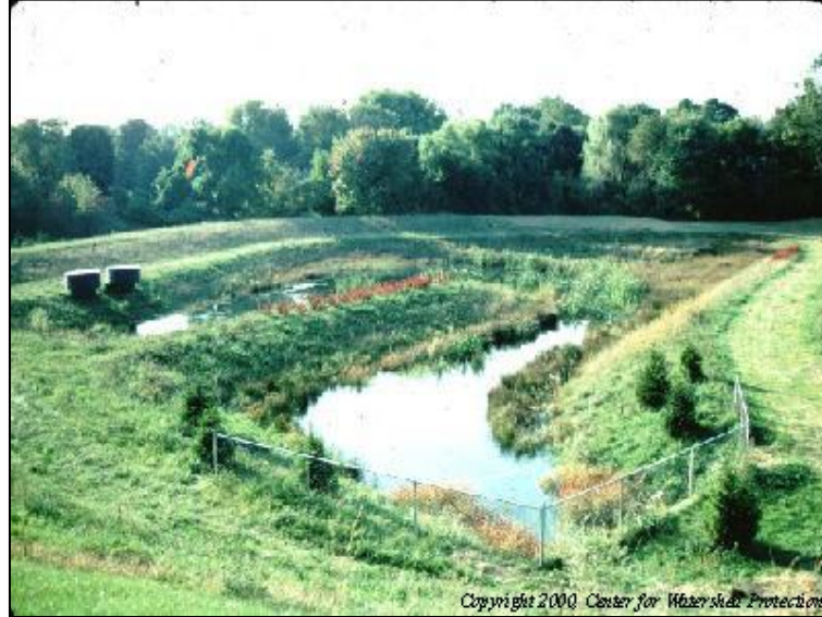
Figure PTP-03- 7 Extended Detention Shallow Wetland
