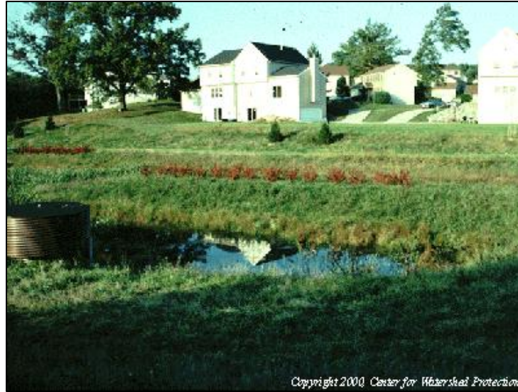
Micropool Extended Detention Pond
