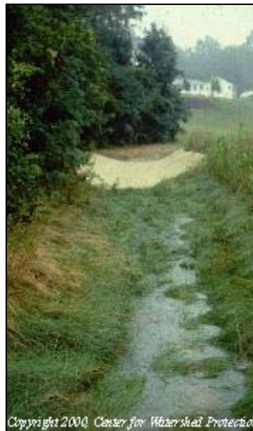
Infiltration Trench
