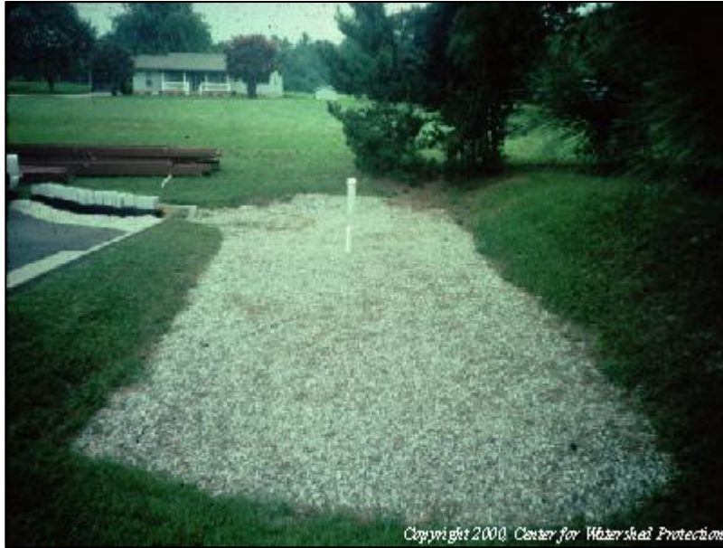
Infiltration Trench
