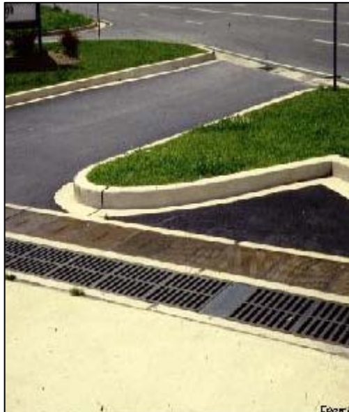
Perimeter Sand Filter
