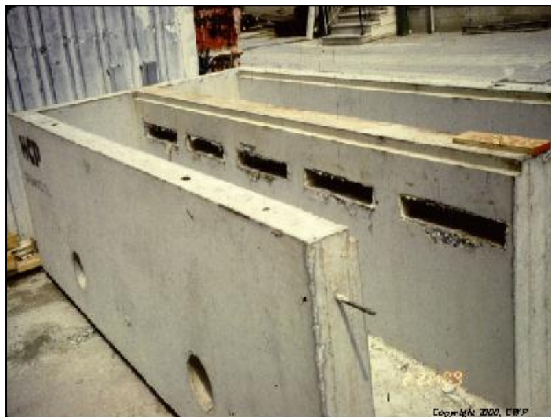
Perimeter Sand Filter
